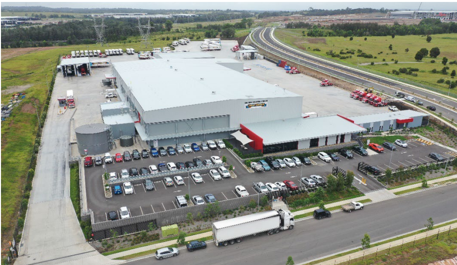
Lindsay Transport Cold Storage Warehouse & Distribution Centre - 55,000m 2
